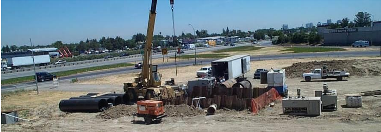
Figure 4. Work Area at Jacking Shaft of Open-Shield Pipejacking Project
