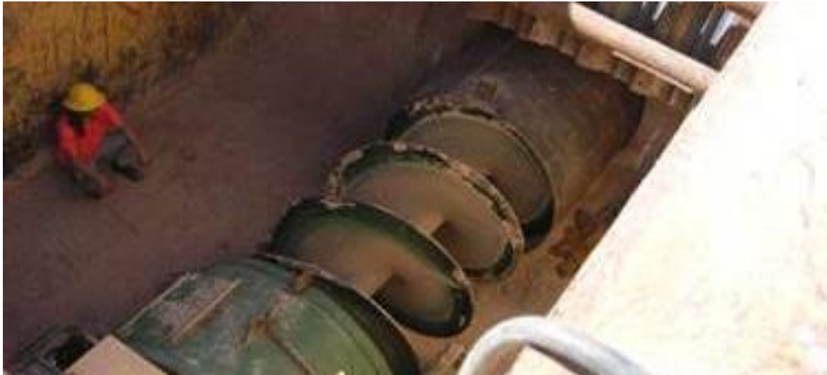
Figure 1. Auger Bore Rig in Shaft Installing Steel Casing
