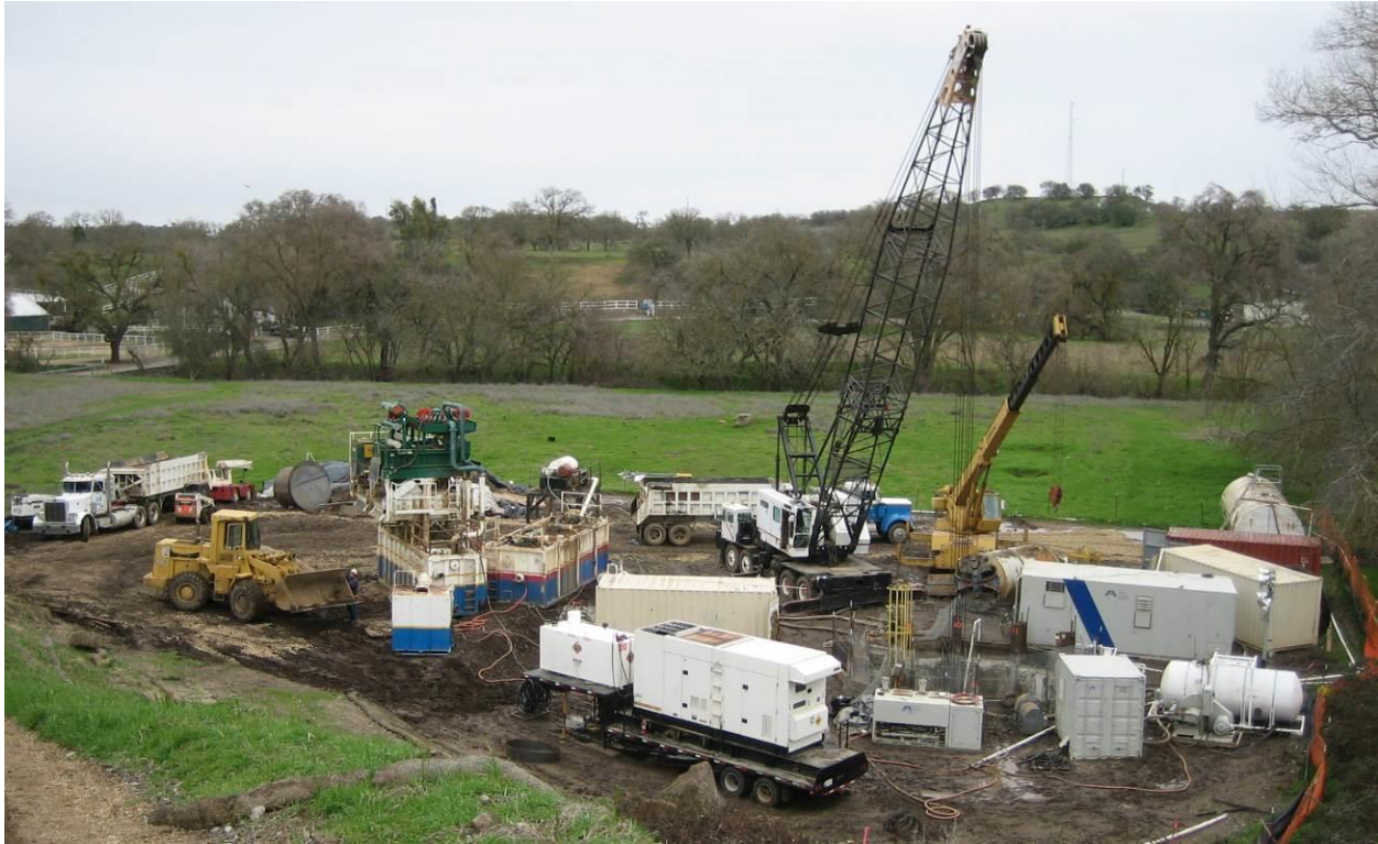
Figure 72. Work Area for Microtunneling Jacking Shaft for 84-inch Concrete Pipe
