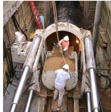
Figure 51. Full Muck Cart in Jacking Shaft
