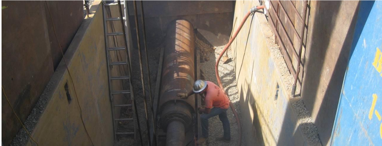
Figure 93. Launch Pit Shored with Trench Boxes for 30-inch Pipe Ram
